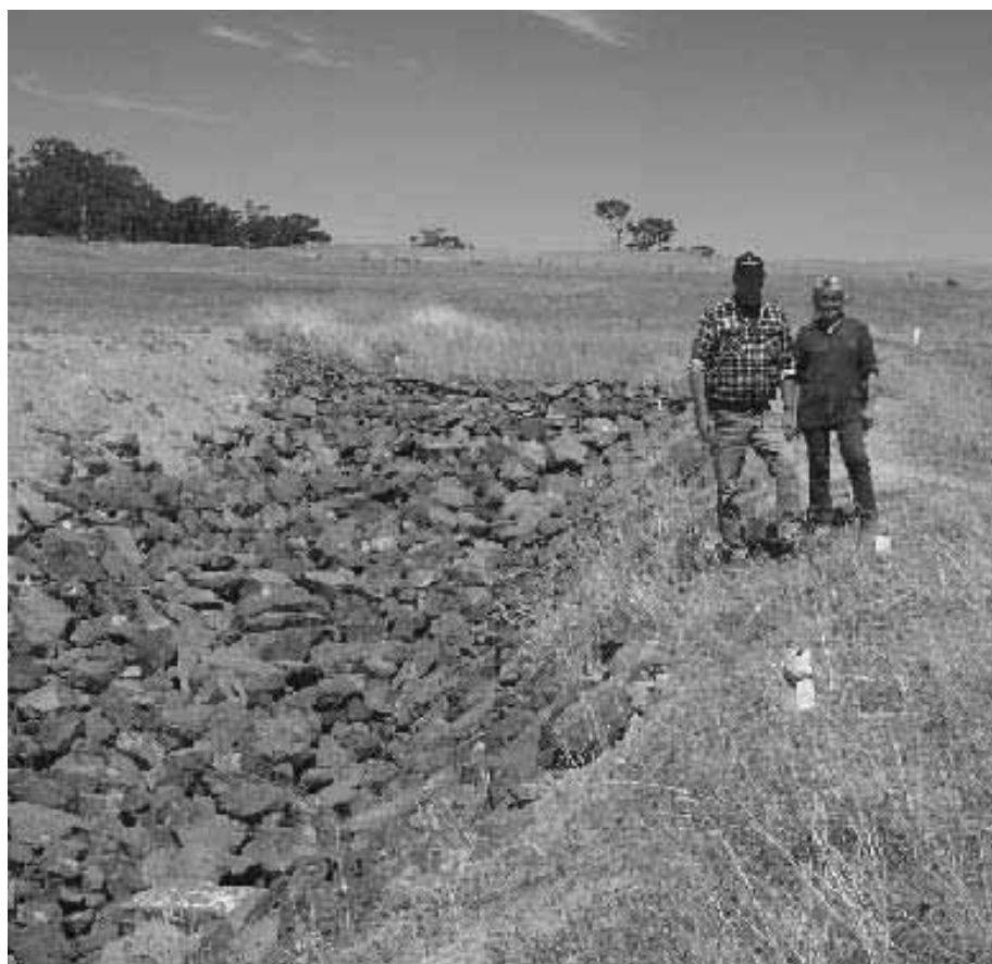
Tony and Glenda Lloyd alongside Racecourse Creek – the rocks have been placed in the creek to halt erosion.
