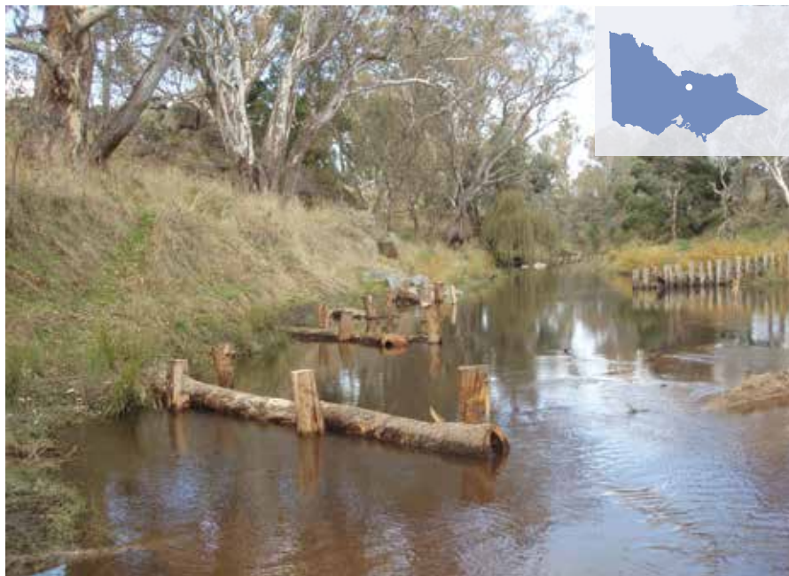
Recycled timber positioned in Seven Creek to encourage bed scour and create greater depth.
