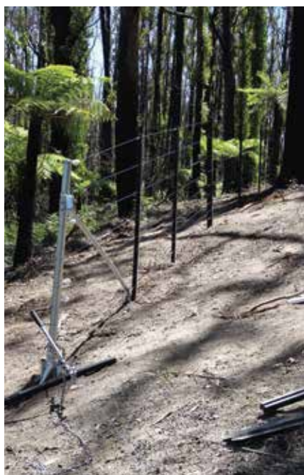
A section of the deer exclusion fence constructed around the fern gully.
