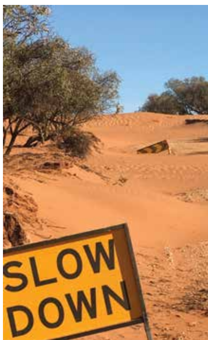
The Karween North Road at Meringur. More than 30 roads were closed in the district during 2019 and 2020 due to sand drift.
