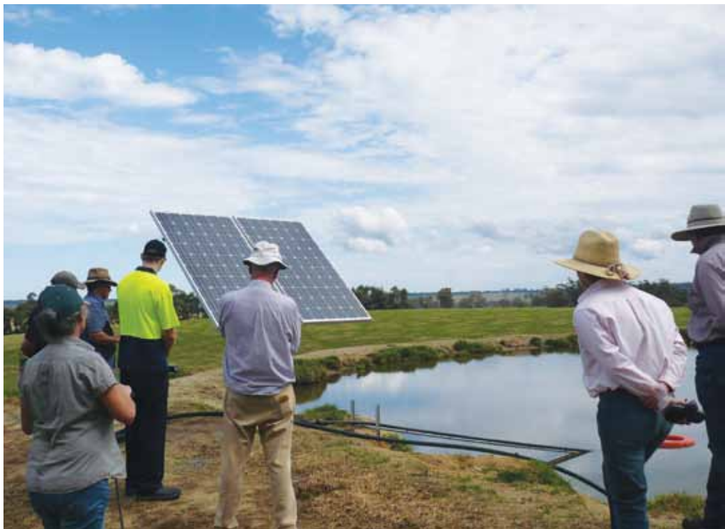
Field day participants inspect a solar water pump on a dam at the Jarrahmond grazing trial site.
