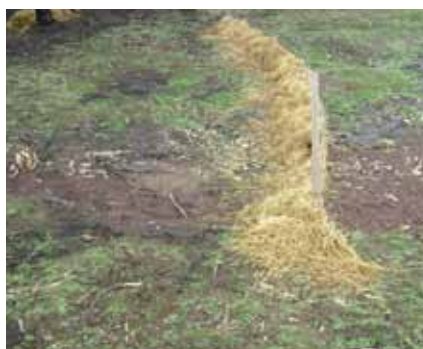
A fairly typical silt trap made from rice straw and old wire not long after installation.
